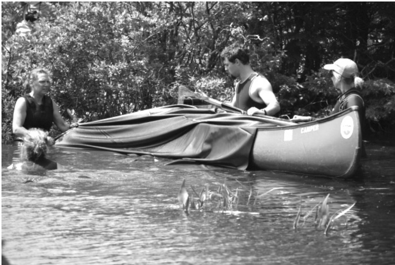
Garrison Beck, DLWA Senior Program Manager, and members from the DEP installing the pond liner.
